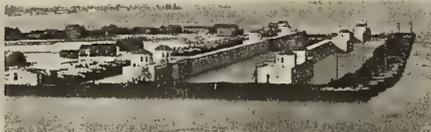
Completed lock ready for withdrawal of piling, and at the time the United States Government was testing the tightness of lock gates, preparatory to acceptance.
